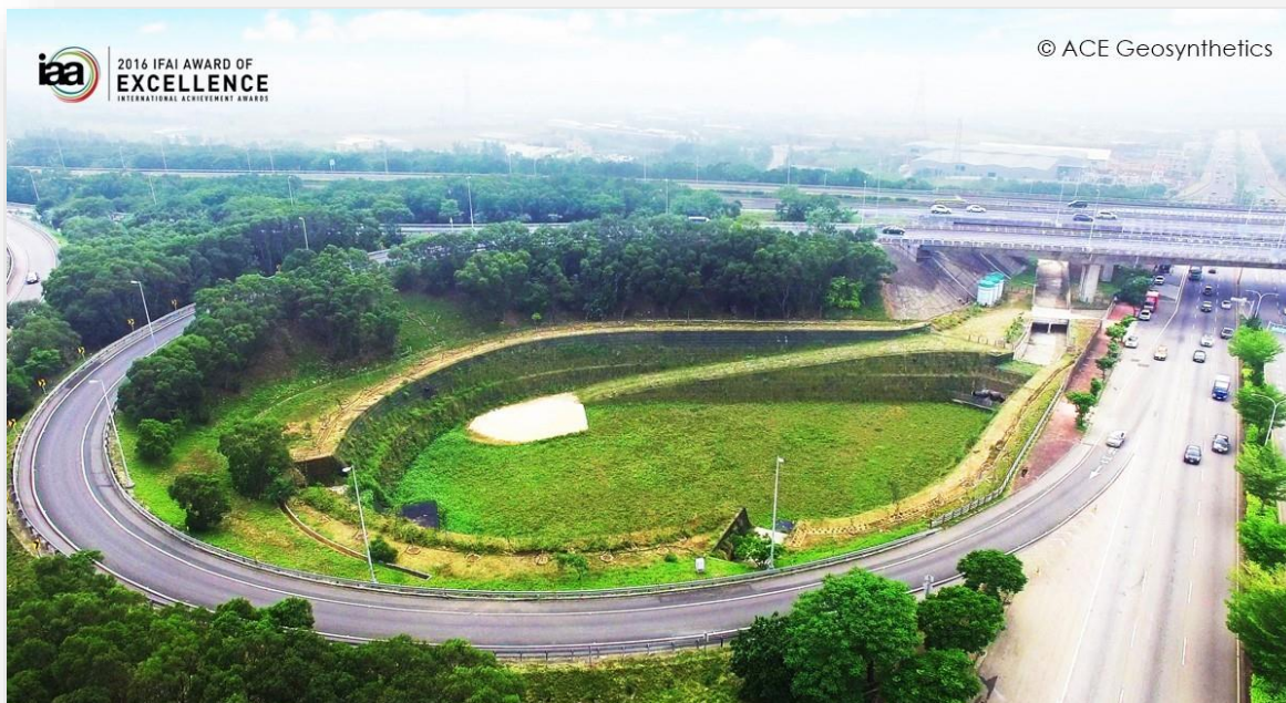
Figure 1. Example of a Detention Basin inside a Loop Ramp
